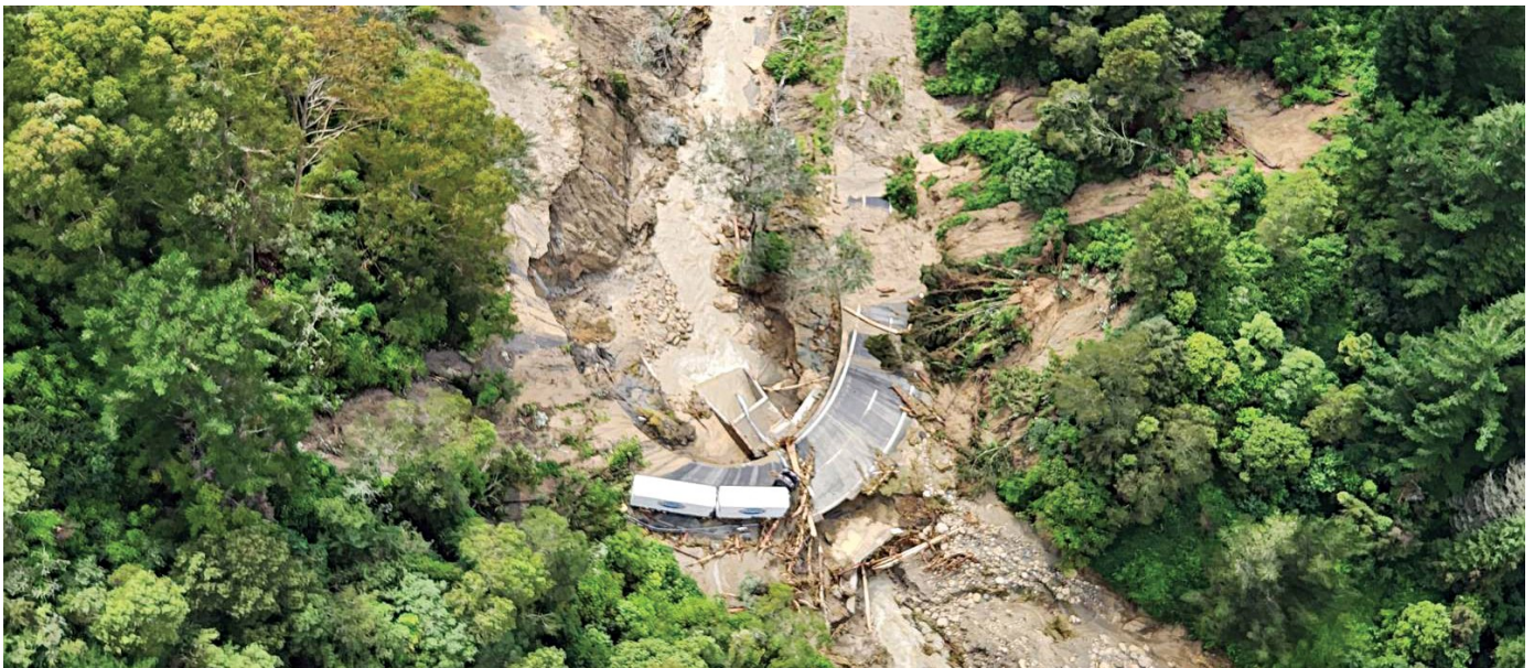
Damage to SH2 between Napier and Wairoa caused by Cyclone Gabrielle [Image: NZDF]
